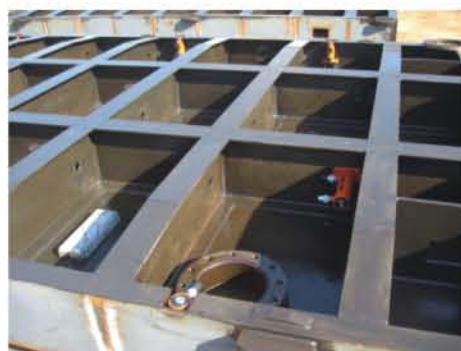
56 ED-308 used in a power generation plant
