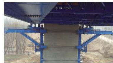
400 ton EAGLE PRO EL series hydraulic cylinders used in bridge building
